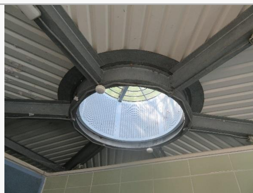
Photo 2: Good view of the roof material and vent.
