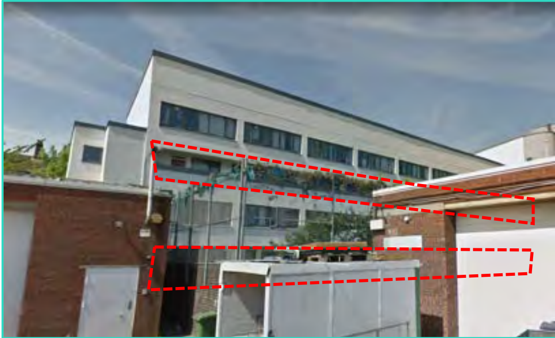
Google Streetview of rear elevation of 142-192 Thessaly Road
