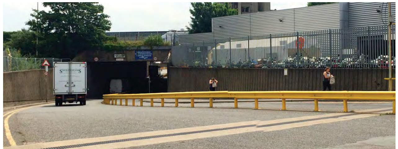
Site Boundary with Raised Rail Tracks - looking South
