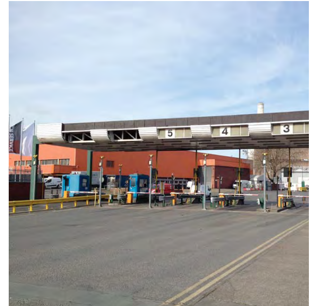
7. View looking from the Covent Garden Market site through the gantry
