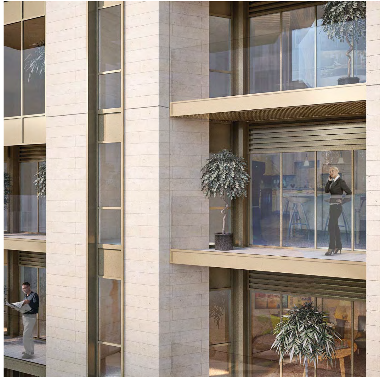
View showing the chamfered balcony detail in bronze metal window frames
