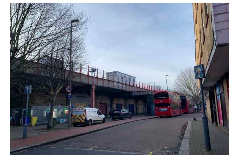
Station approach from north east
