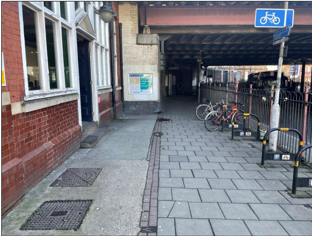
Photograph 9: Sheffield Stands outside Queenstown Road Rail Station along Route 2
