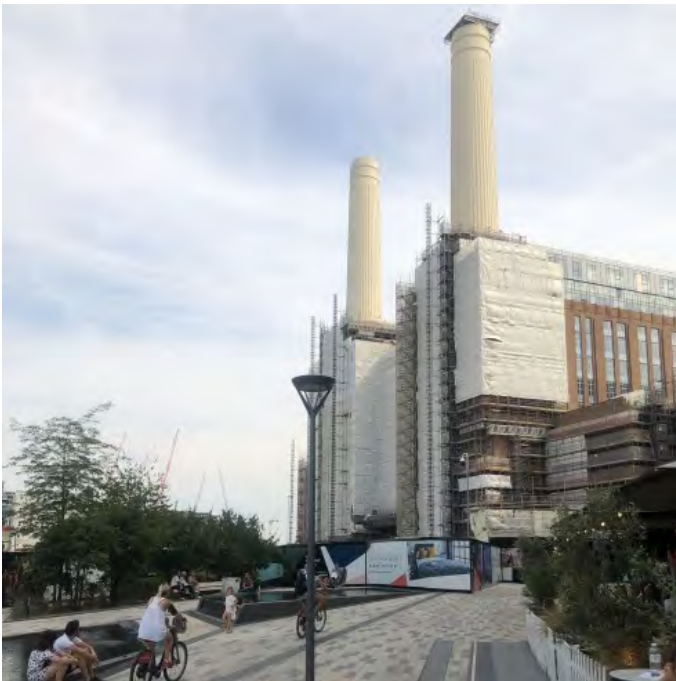
Picture 5.4 The iconic Battersea Power Station during redevelopment
