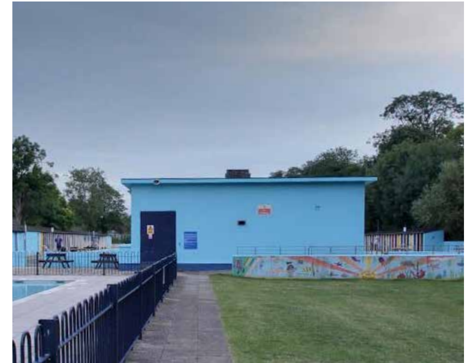
2. Rear of the existing café building
