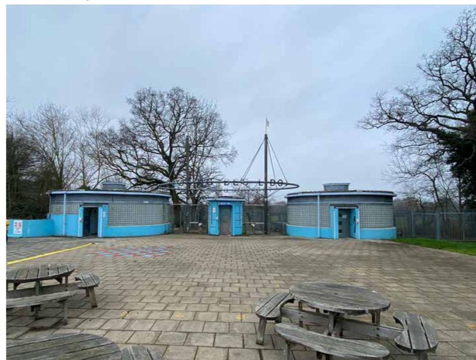
3. Existing entrance and changing facilities and paved area
