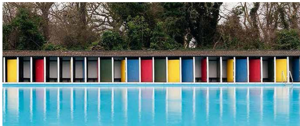
Timber Colonnades Between Cubicles
