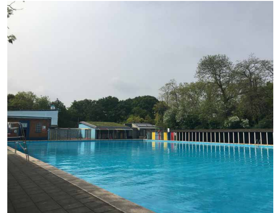
2. Looking south towards the pump room and pavilion
