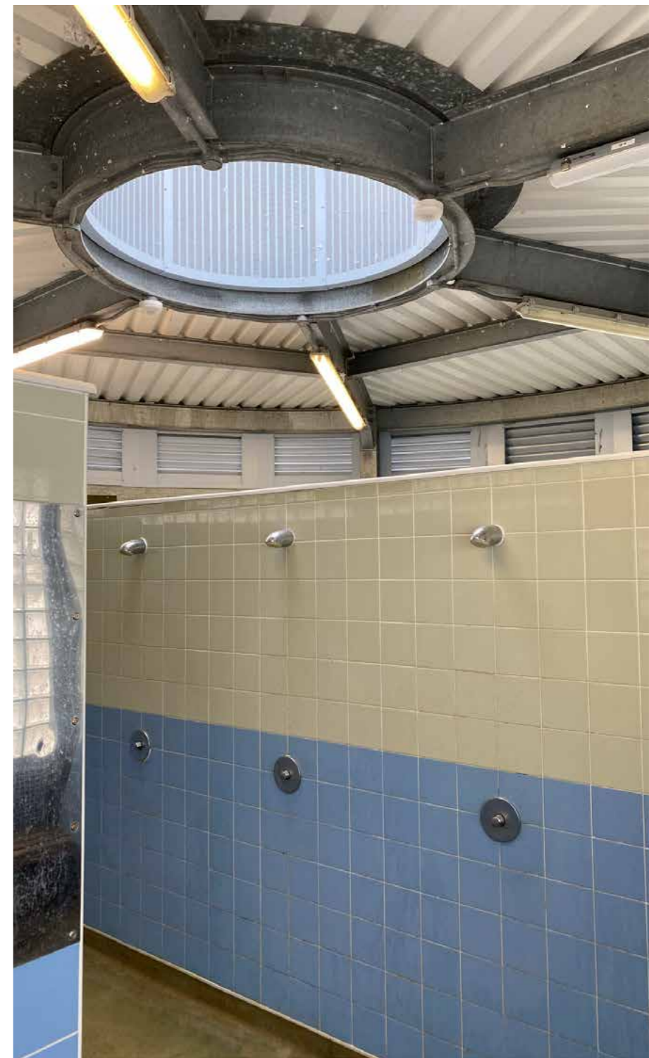
2. Condition of the existing showers
