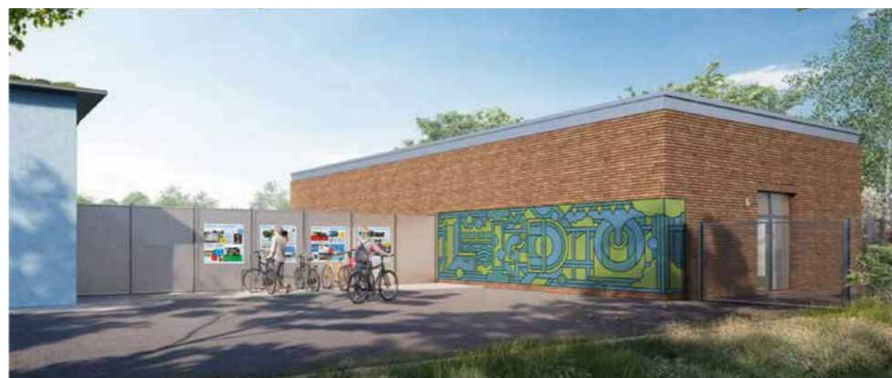
Solid Rear of the Pump House
