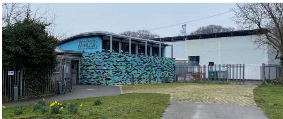
Solid Rear of the Pavilion
