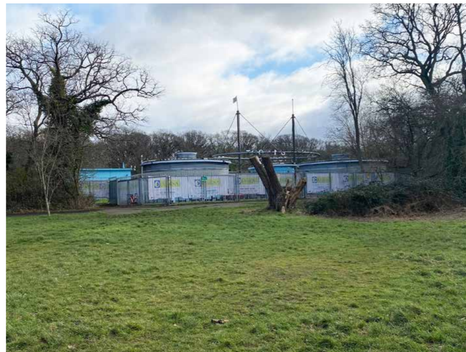
1. The existing entrance from the Common
