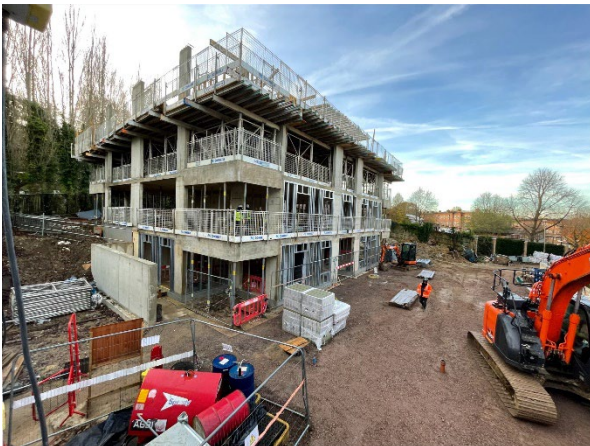
Metal façade install
