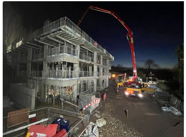
Pumping concrete to the third-floor columns and stair core
