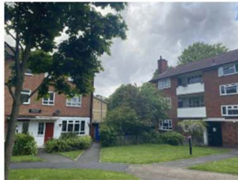
3. Site view looking North-West
