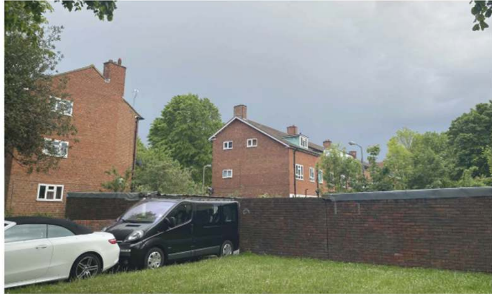
2. Site view looking South-East
