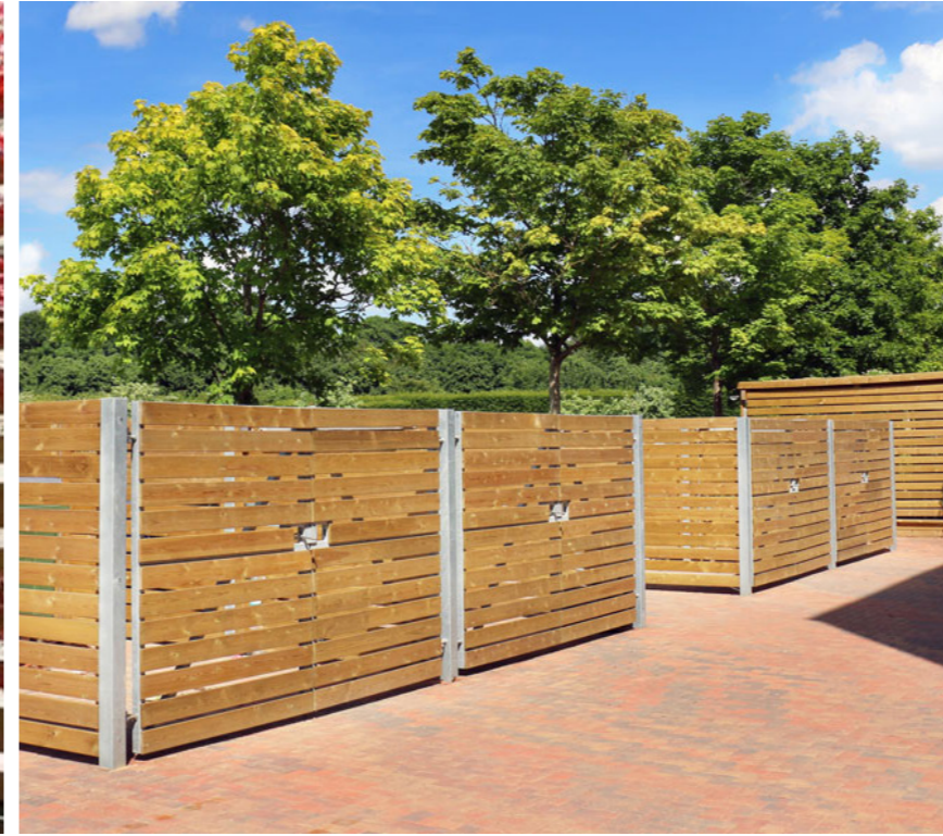
Bins and bikes storage enclosure
