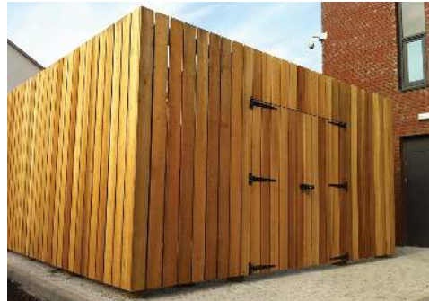
Enclosed bin storage example
