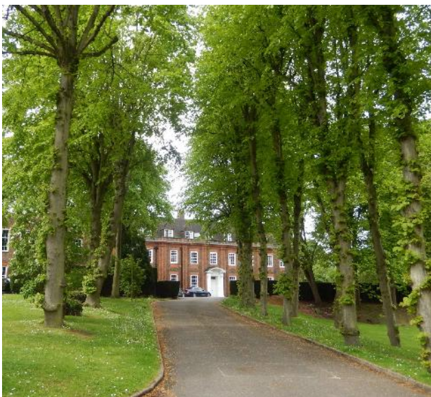
Picture 9.1 Kairos Centre, a locally listed building, situated within acres of landscaped gardens and overlooking the historic Richmond Park
