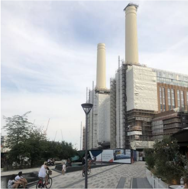
Picture 5.3 The iconic Battersea Power Station during redevelopment
