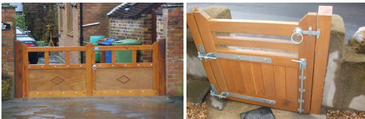
Figure D-3 Example of flood gates
