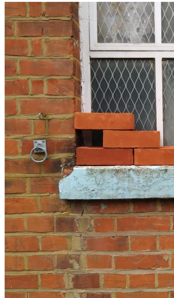
Proposed bricks in light red compared with existing bricks
