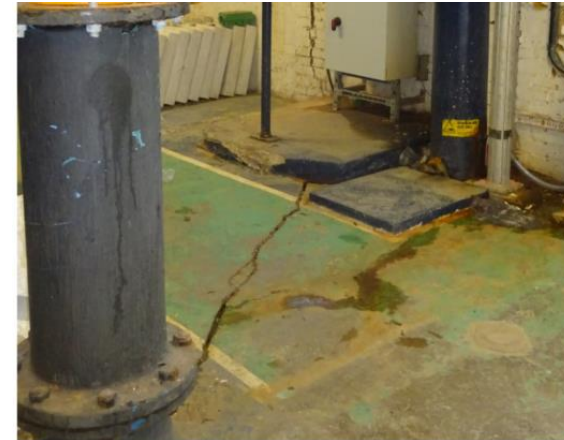
Slab crack
