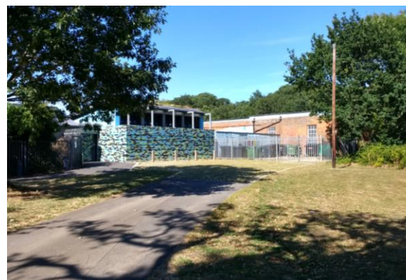
View of the new pavilion from the parking area with the pump house on the background
