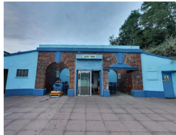
South entrance arches prior to demolition
