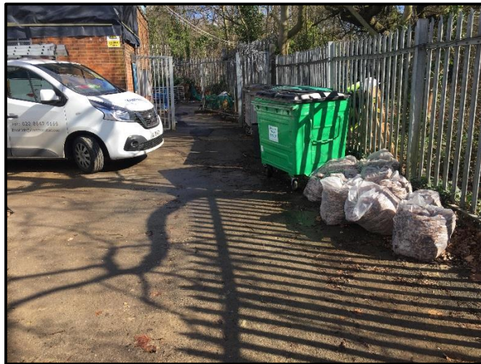
Photo 4.1: Hard-standing to the west of the existing pump house.
