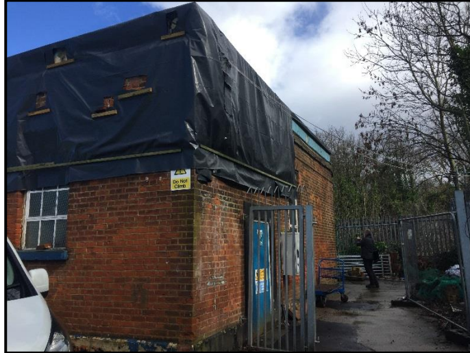
Photo 4.6: Pump house, south western elevation.
