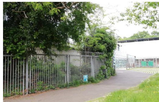
Existing fence surrounding the pavilion
