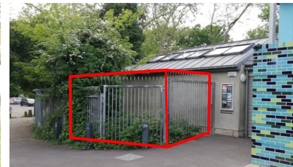
Entrance of the pavilion. The red line indicates the approximate location of the proposed substation
