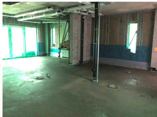
Screed to all duplex flats complete
