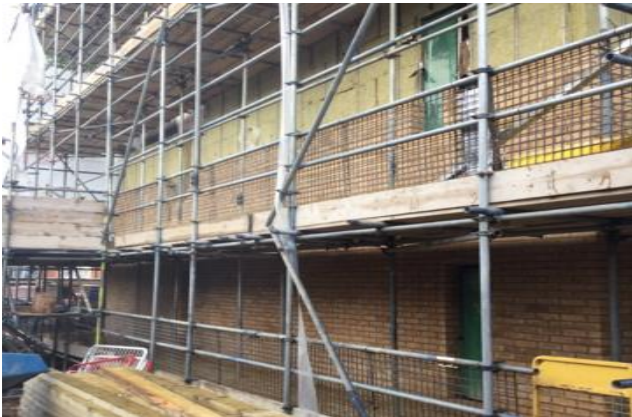
Level 2 decking – SFS, insulation, brick channels complete, all windows fitted
