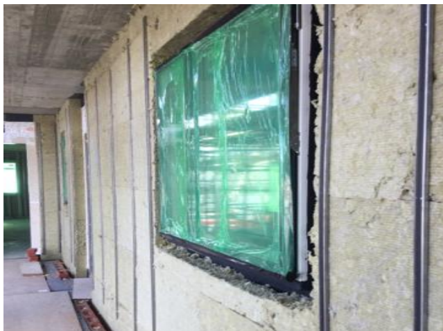
Level 2 decking – SFS, insulation, brick channels complete, all windows fitted
