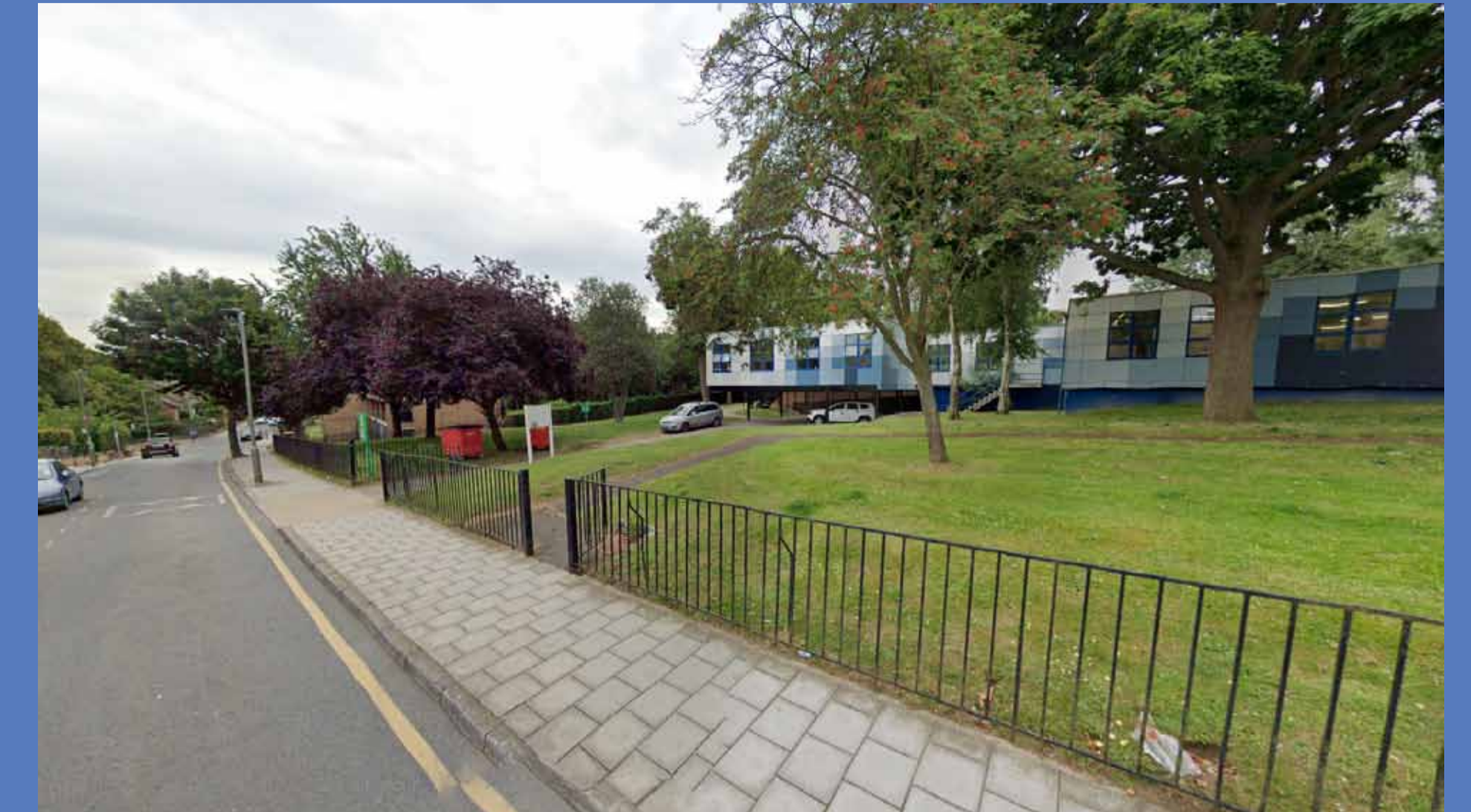
Street view of the existing building
