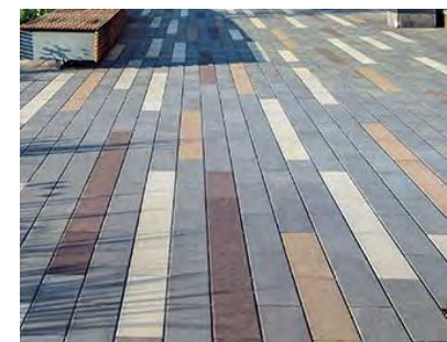
Area A Paving to entrance areas
