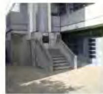
V1. Chute and building entrance
