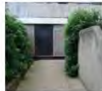
V2. Access to Storage / Falt
