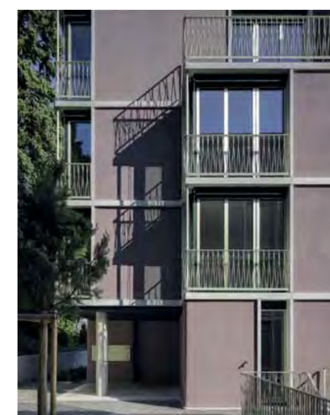
Framed metal balconies within an exposed frame.
