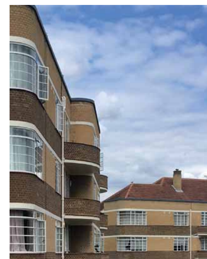
Local context showing strong contrasting brick colours.
