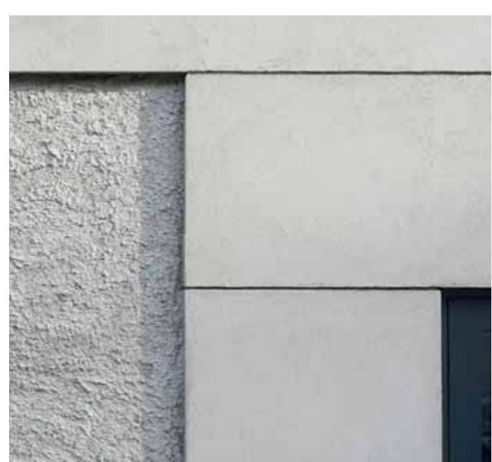
Inset textured panels to exterior.
