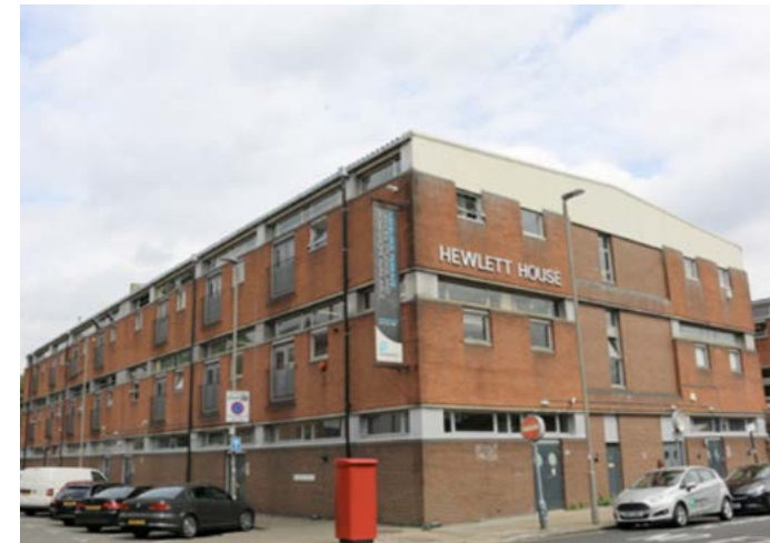
Hewlett House hosts different types of creative activities such as lighting design, graphic design and fabric & clothes manufacturing
