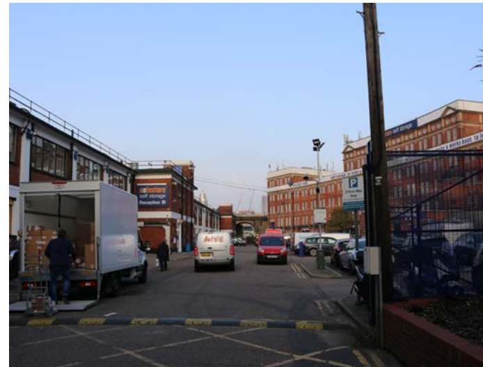
Open space at the Safestore site is currently used as a parking space and a loading area. Potential to create shared yard space and amenity space for the employees and the visitors
