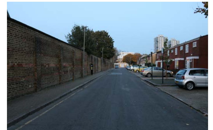
Gatwick Express depot site obscured by a perimeter wall creating inactive frontage. Tree screening and pavement improvements needed to create a more pleasant route to Heathbrook Park.
