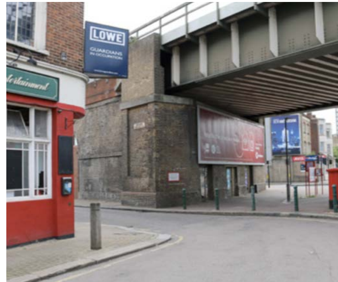
Unwelcoming entrance from Battersea Park Rd. Non-inclusive design due to the level change, pavement improvements needed.
