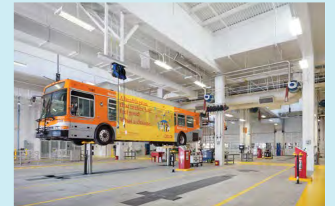
Bus operations and maintenance facility MTA Division 13, Stantec
