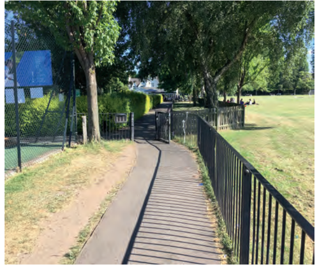
Figure 20: Fencing pinch point at Skylark Cafe and tennis courts
