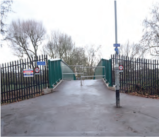
Figure 7: Cycling signage at Cats Back Bridge
