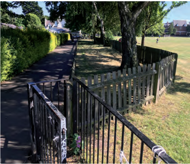
Figure 21: Fencing pinch point at Skylark Cafe and tennis courts
