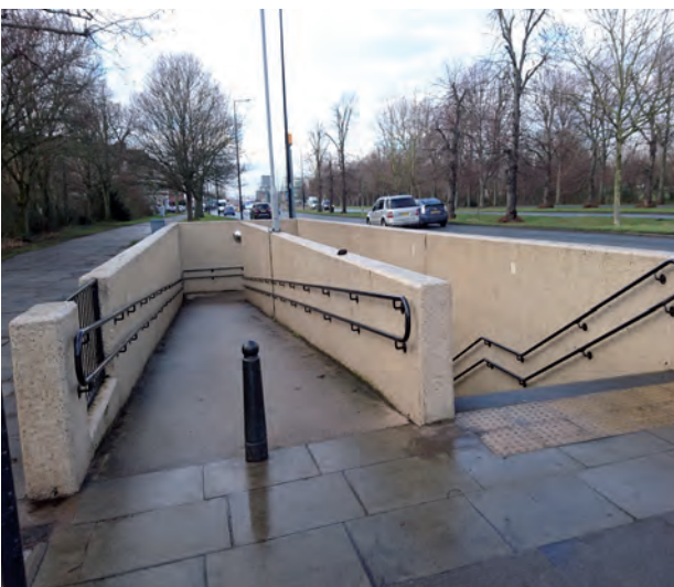
Figure 23: Underpass under Trinity Road between Westside and Northside Field
