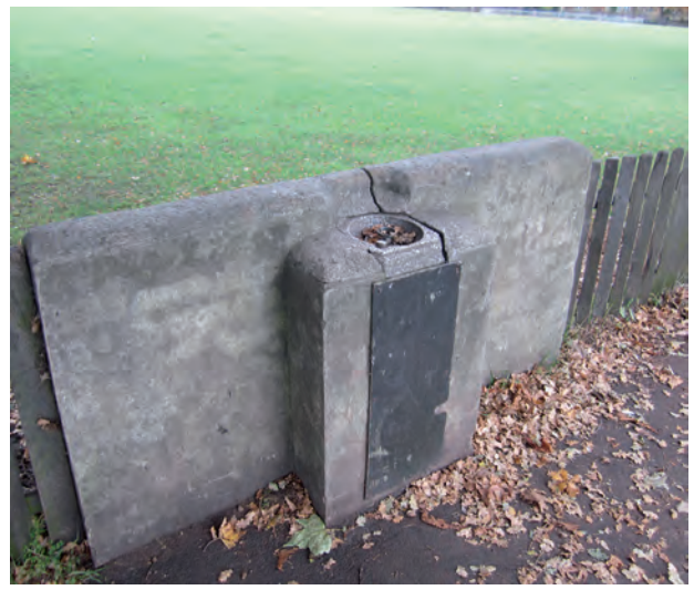
Figure 16: Out of use water fountain, Skylark Cafe
