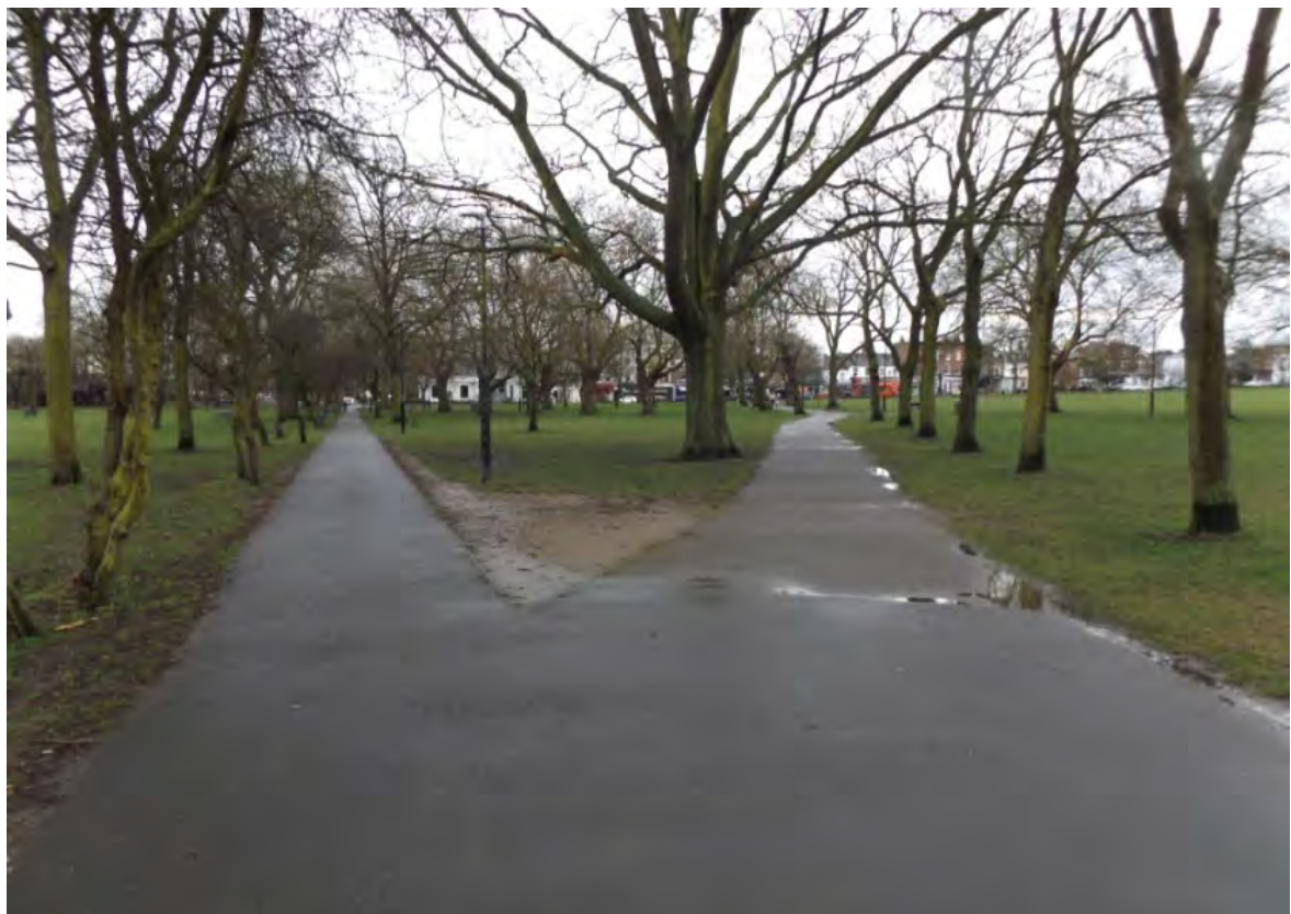
Figure 7.9 Footpaths near Bellevue Road showing typical marginal conditions
