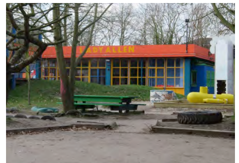
Lady Allen building exterior
