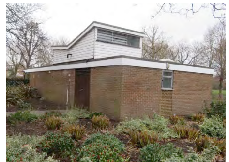
Nursery from south
