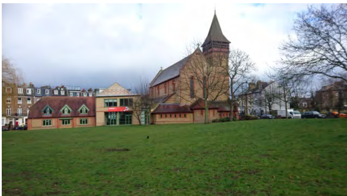
View from footpath crossing eastern section of St Mark's Area
