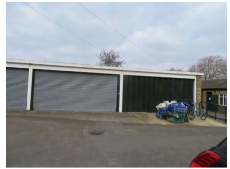
Garages from south
