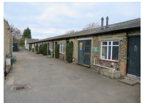
East range from south
