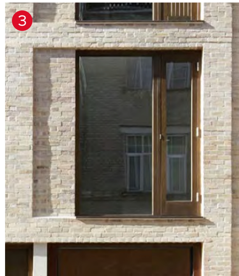
Windows & recess brick
