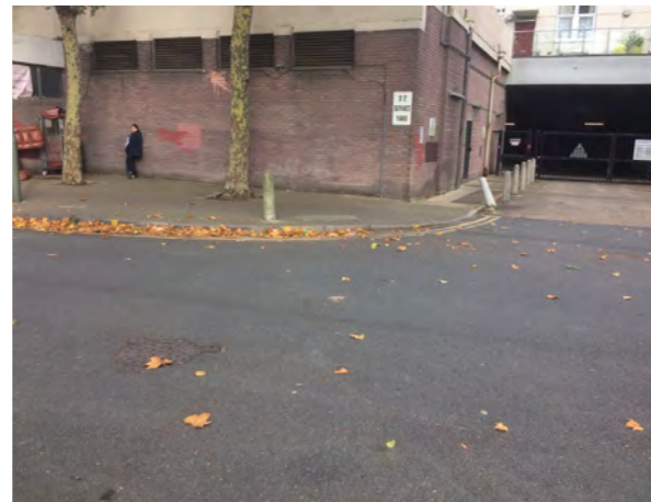
E16 entrance - poor dropped kerb provision
