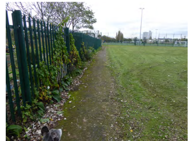
Route 6 - poor maintenance (slip hazards with moss growth)
