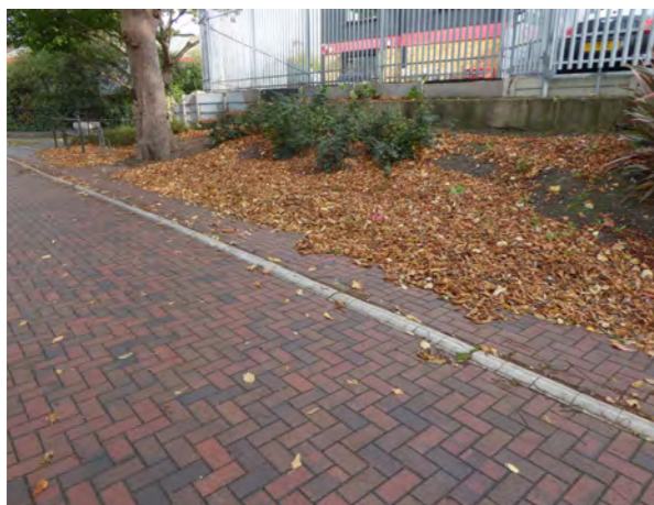
Route 1 - cycle path narrows - poor maintenance
