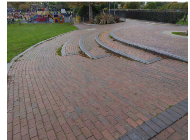
Route 1 - no tactile warnings for feathered steps and contrast poor on nosings
