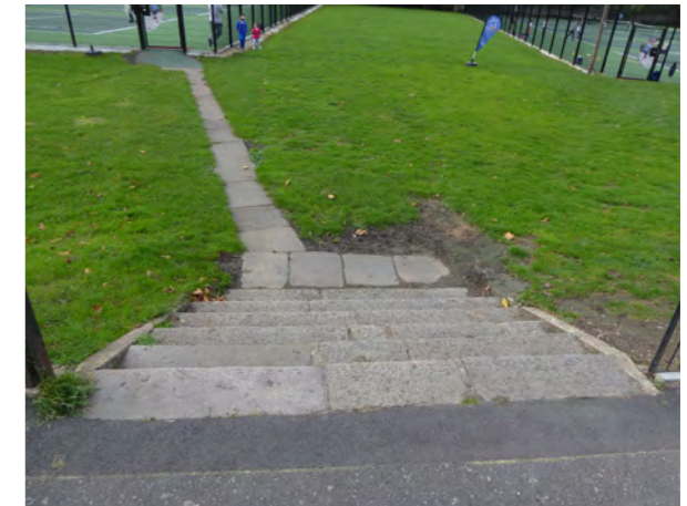
Route 1 - tennis courts - no handrails, contrasting step nosings or tactile paving
