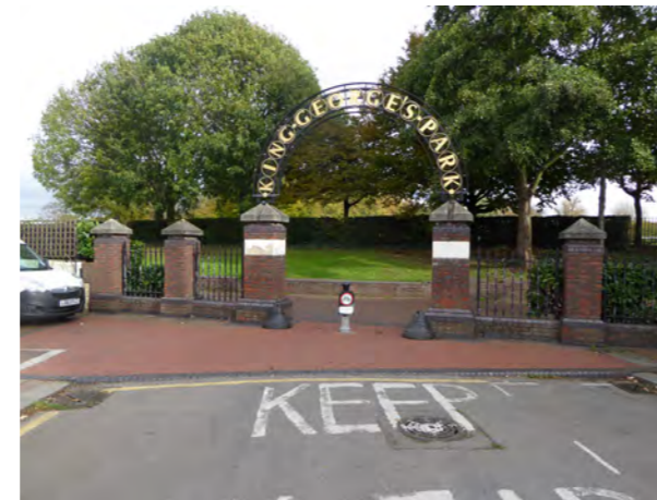
E9 entrance - low level bollards
