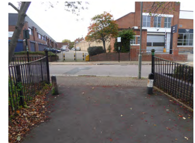
E6 entrance - lack of dropped kerbs
