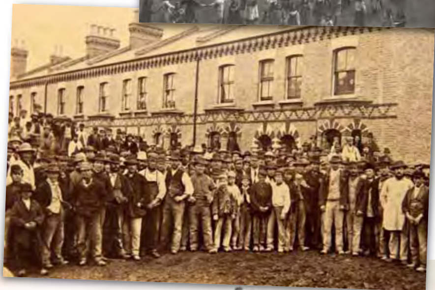
Building workers construct the Shaftesbury Park estate
