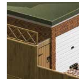
Locked side gate, not recessed
