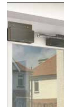
Communal door with magnetic lock and automatic closer
