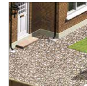
Gravel driveways and paths
