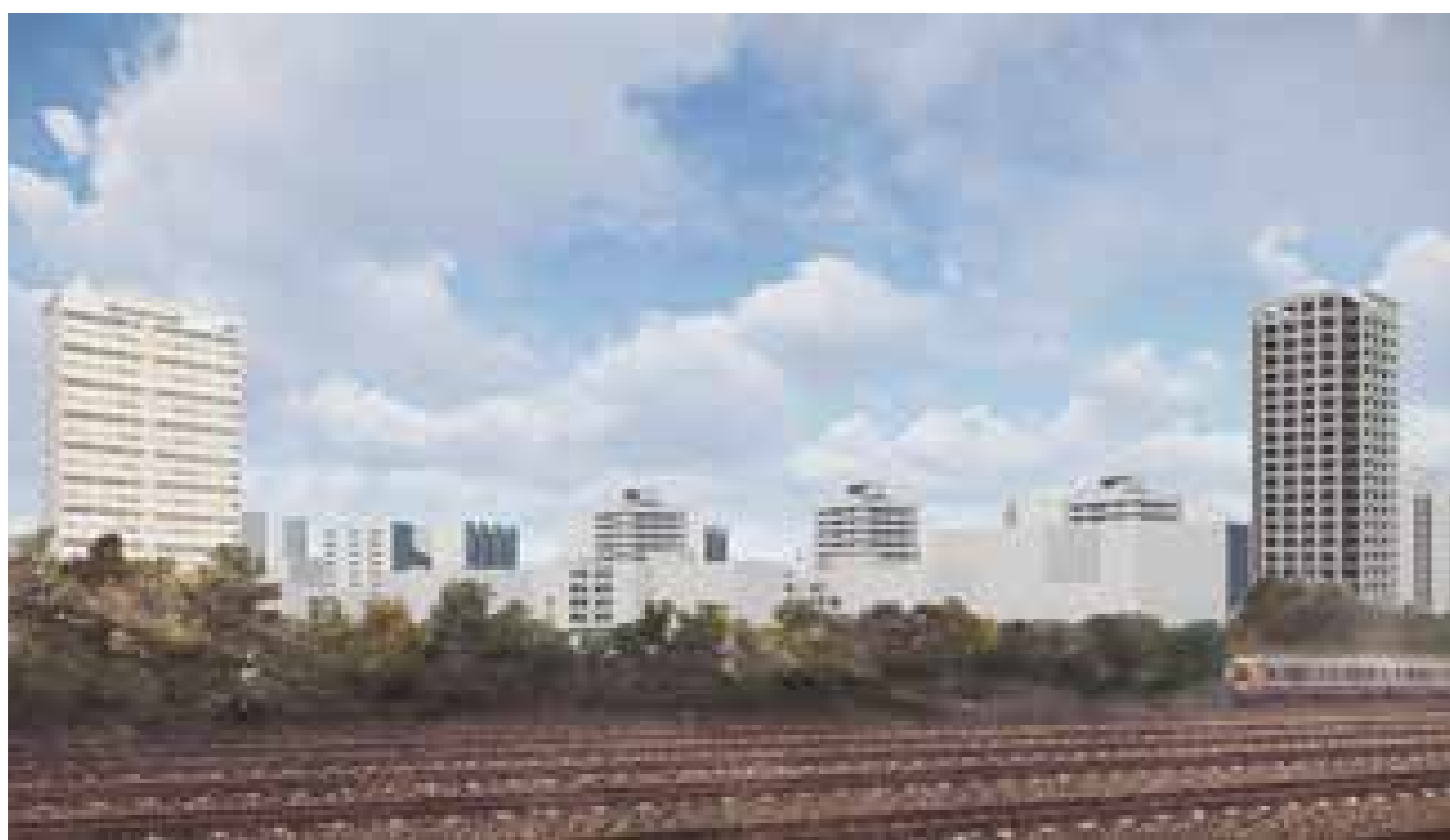
View across Railway
