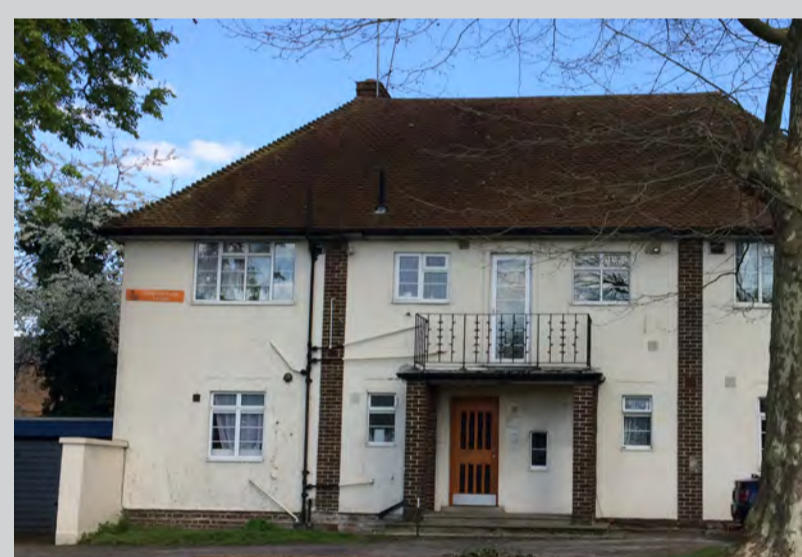
3 Sherwood Lodge to be demolished
