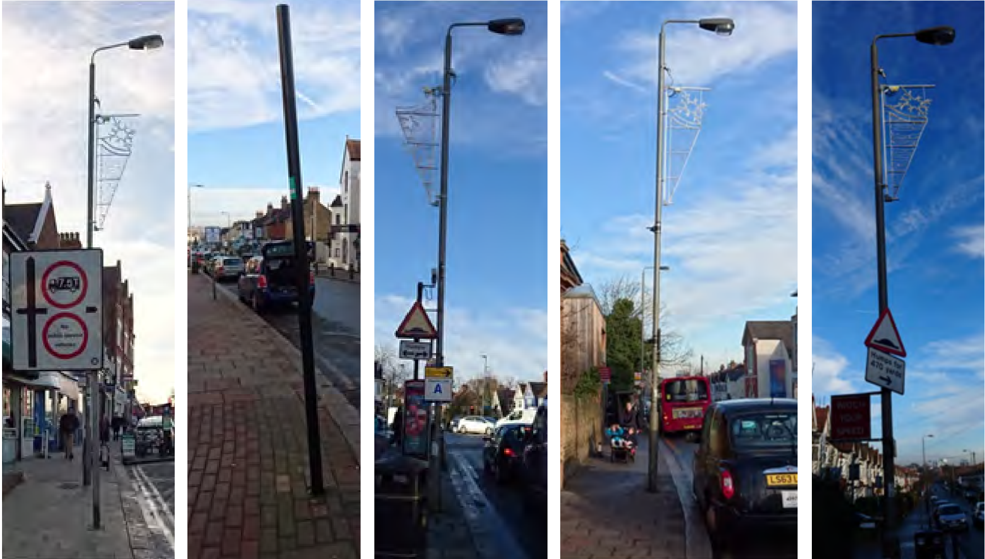
Existing columns and street furniture
