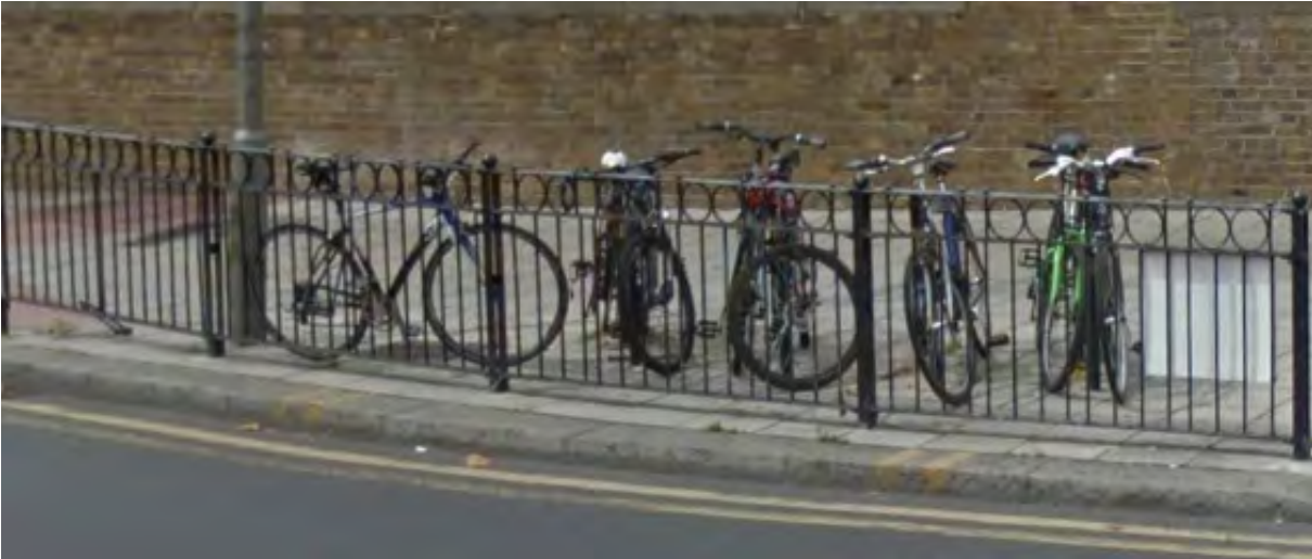
Existing guardrails / bike stands by the station
