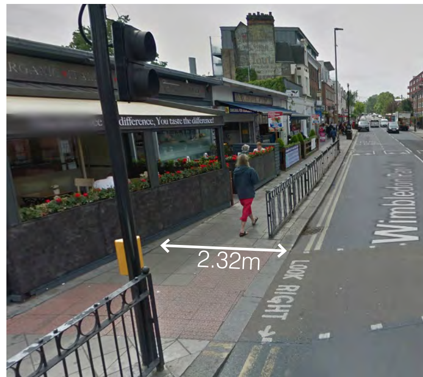
Existing pinch point at Wimbledon Park Road (south)
