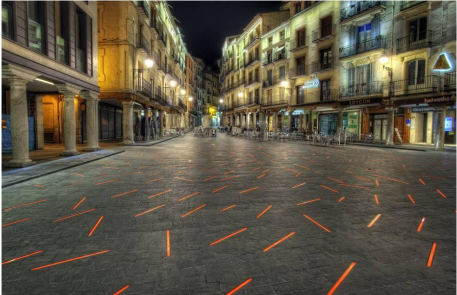
Figure 8 - Linear strip lighting
