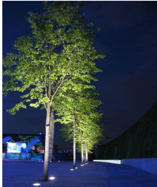
Figure 10 - Recessed tree up lighters
