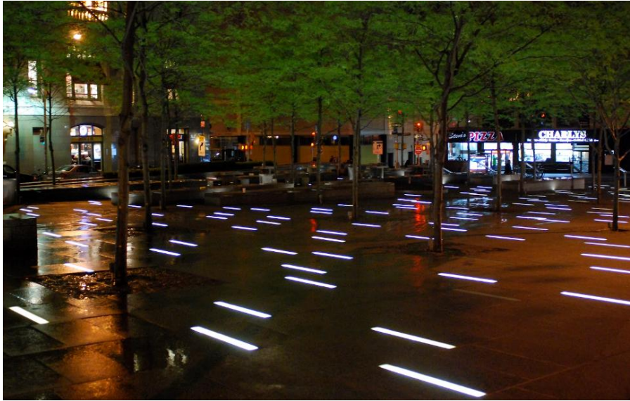
Figure 9 - Linear strip lighting
