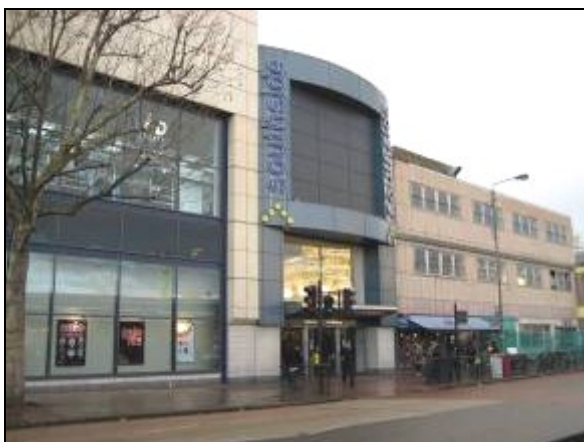
View of entrance to Southside Shopping Centre from Garratt Lane
