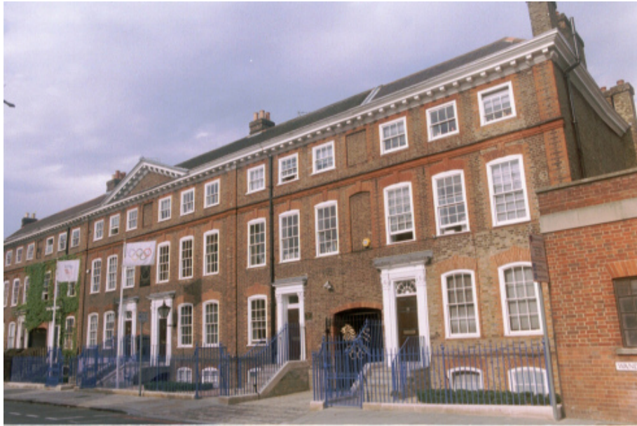
Picture 8.6 1-6 Church Row, Wandsworth Plain, SW18 (grade II*)
