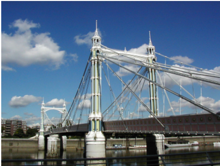
Picture 8.7 Albert Bridge, Albert Bridge Road, SW11 (grade II*)
