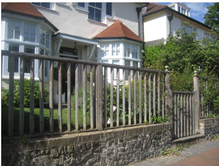
Figure 23 : Reinstated original style boundary wall and fence at 13 Rodway Road
