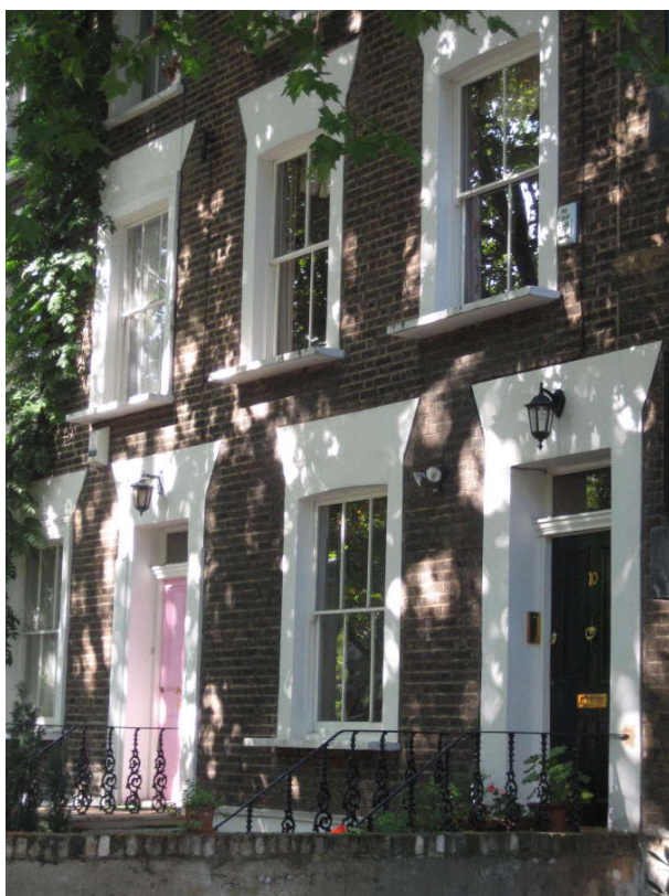
Picture 4 Westbridge Road
