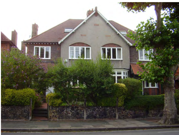
Figure 82 : Original wall made of kiln-burnt bricks
