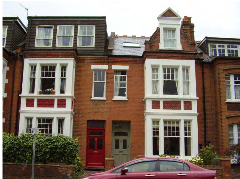
Figure 35 : Nos. 9-11 showing the shocking difference between the original gabled dormer and the mid 20th century ones
