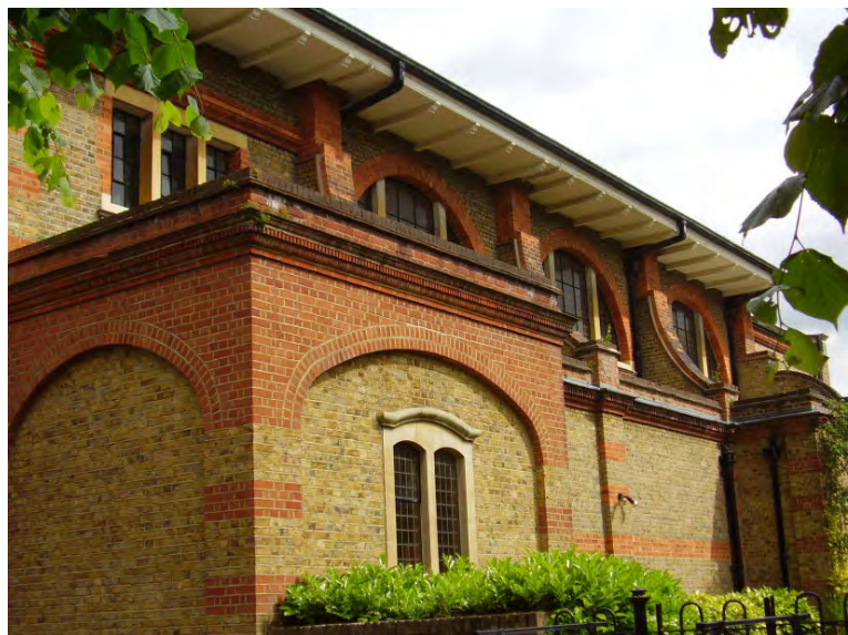
Figure 56 : Diocletian windows and overhanging eaves at Our Lady of Pity and St Simon Stock
