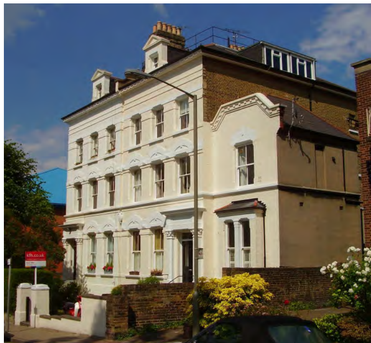
Figure 93 : Belgravia Villas, 5-6 Burston Road
