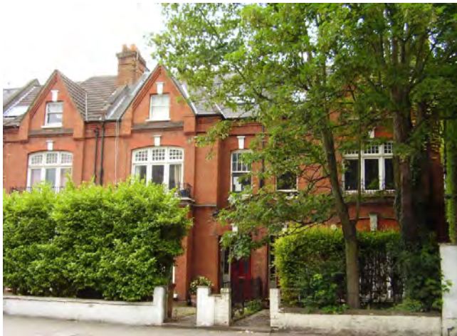
Figure 36 : Red brick terrace at nos. 263-269
