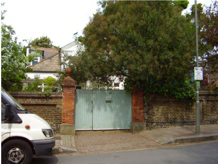
Figure 119 : Original wall and gate piers on Cambalt Road
