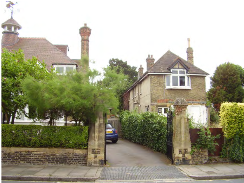
Figure 83 : Wall and gate piers at 1c Luttrell Avenue
