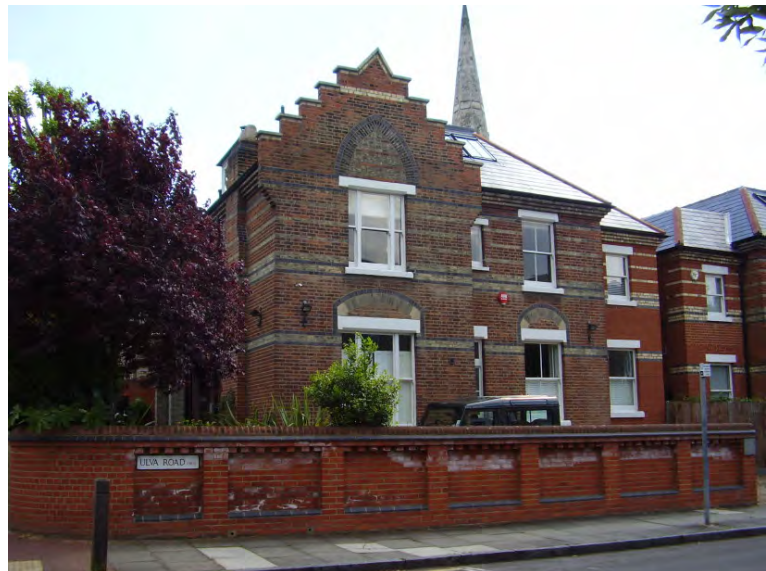
Figure 103 : Rebuilt polychromatic brick wall in Ulva Road
