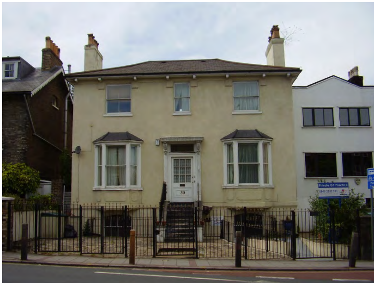
Figure 120 : Unsympathetic modern railings to 30 Putney Hill
