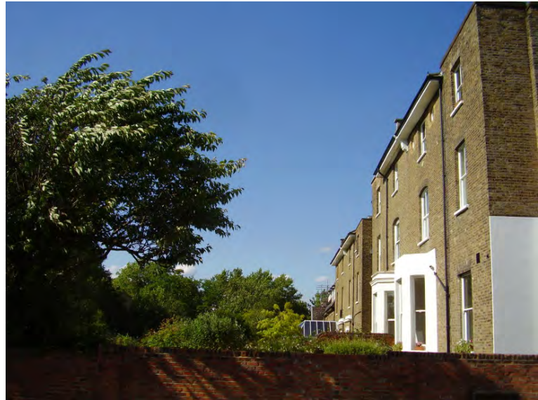
Figure 92 : Clearly visible rear elevations and long gardens
