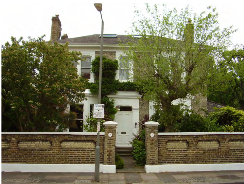
Figure 42 : Stock brick wall at 7 Malbrook Road
