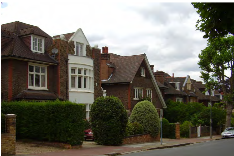
Figure 58 : St. Simon's Avenue with no. 12 in the foreground and no. 10 with its sweeping catslide roof to the right
