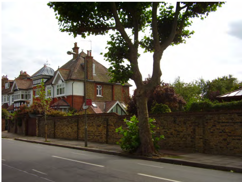
Figure 84 : Traditional stock brick wall to the rear garden of 3 Genoa Avenue
