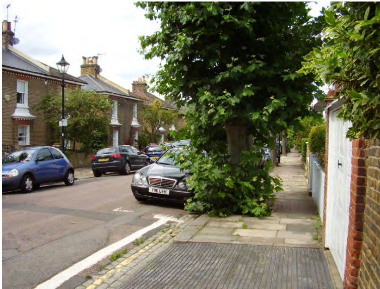
Figure 85 : Scorria blocks on Coalecroft Road. The traditional (albeit small) paving slabs can also be seen.
