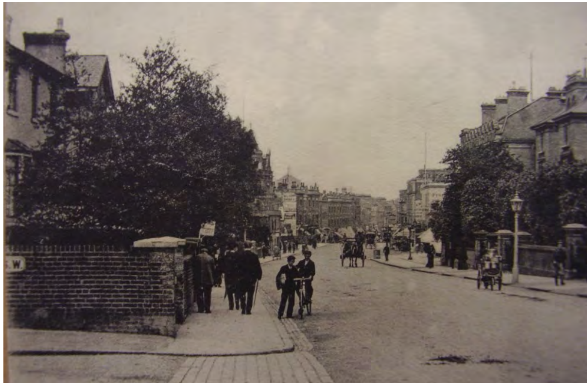
Figure 9 : Looking south down Putney High Street
