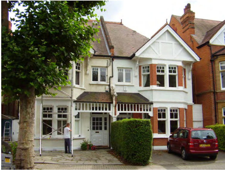
Figure 89 : Full width hardstandings without any landscaping or front boundary are harmful to the leafy character of the conservation area
