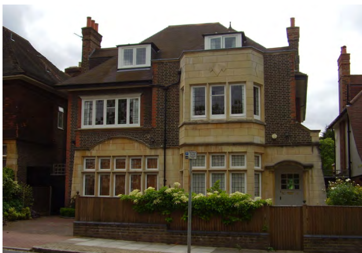
Figure 61 : Original style fence on low brick wall in St. Simon's Avenue
