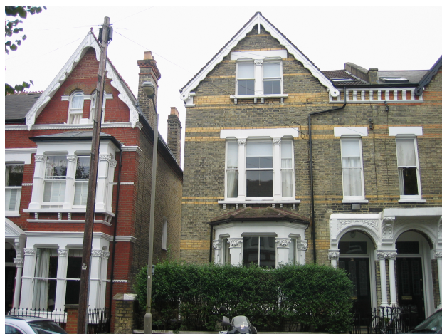
Picture 5 Notice the ornate barge boards
