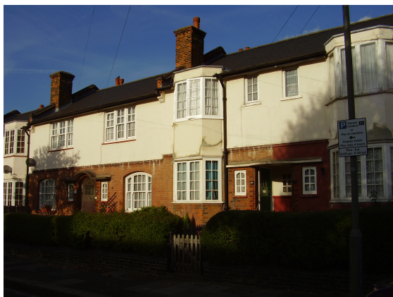
Picture 1.5 Terrace of cottages constructed of yellow stock brick with roughcast render on the upper storey
