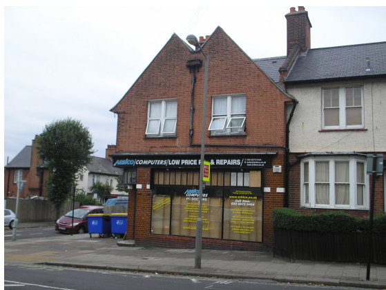
Picture 2.1 Original shopfront in need of repair
