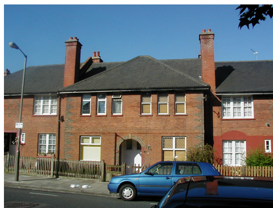
Picture 2.2 Replacement windows take away from the special character of the terrace
