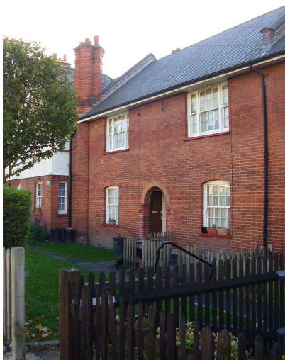
Picture 1.7 Timber sliding sash windows with georgian glazing bars
