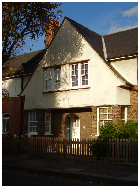
Double pitched front gabled roof in the middle of a terrace
