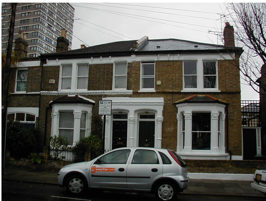
Figure 2 The paint has been removed and the appearance of one larger house or villa has been restored
