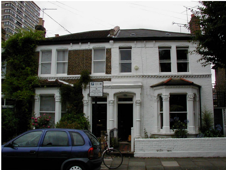
Figure 1 The painting on this semi-detached house disrupts the appearance of the pair of houses
