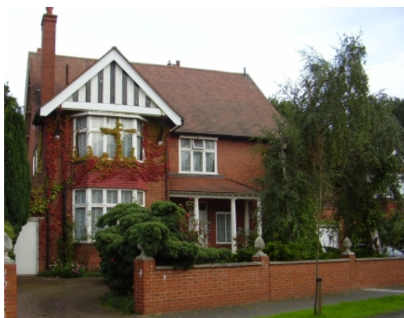
Figure 33 : A 1930s house of remarkably similar design to the one on the right. Its important details include the clay tile roof, applied timbers to the gable, tile hanging to the canted bay, timber framed casement windows, plain red brickwork and open porch.
