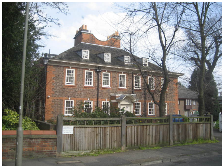
Figure 19 : Yew Tree Lodge, 2 West Drive
