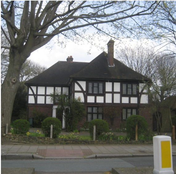
Figure 29 : 2 Ullathorne Road seen from Thrale Road
