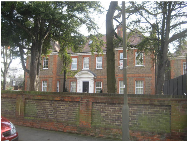
Figure 13 : 5 North Drive with boundary wall
