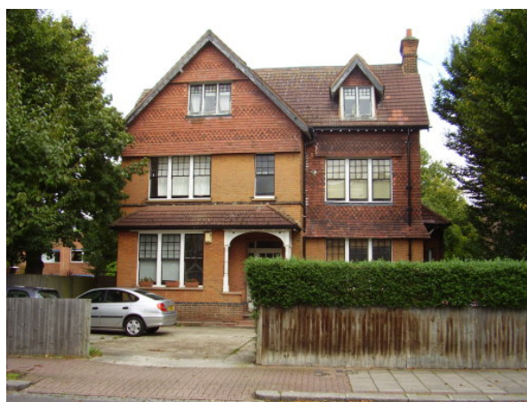
Figure 34 : A house of c.1900 in a typically Edwardian style that would have inspired the house on the left. Original features include clay tiles to roof and facade, nine-over-one paned sash windows and open porch. Original front doors are also extremely important although they are not visible here
