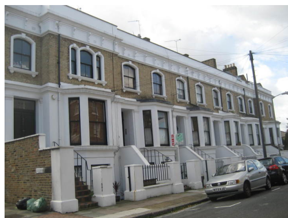
Figure 48 Two storey half stuccoed terraces with basement
