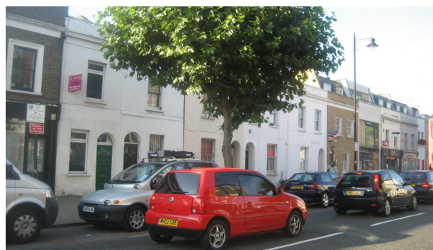
Figure 39 Painted houses at nos. 175-183 St John's Hill
