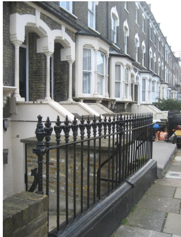
Figure 18 Original railings on a low plinth survive in Cologne Road
