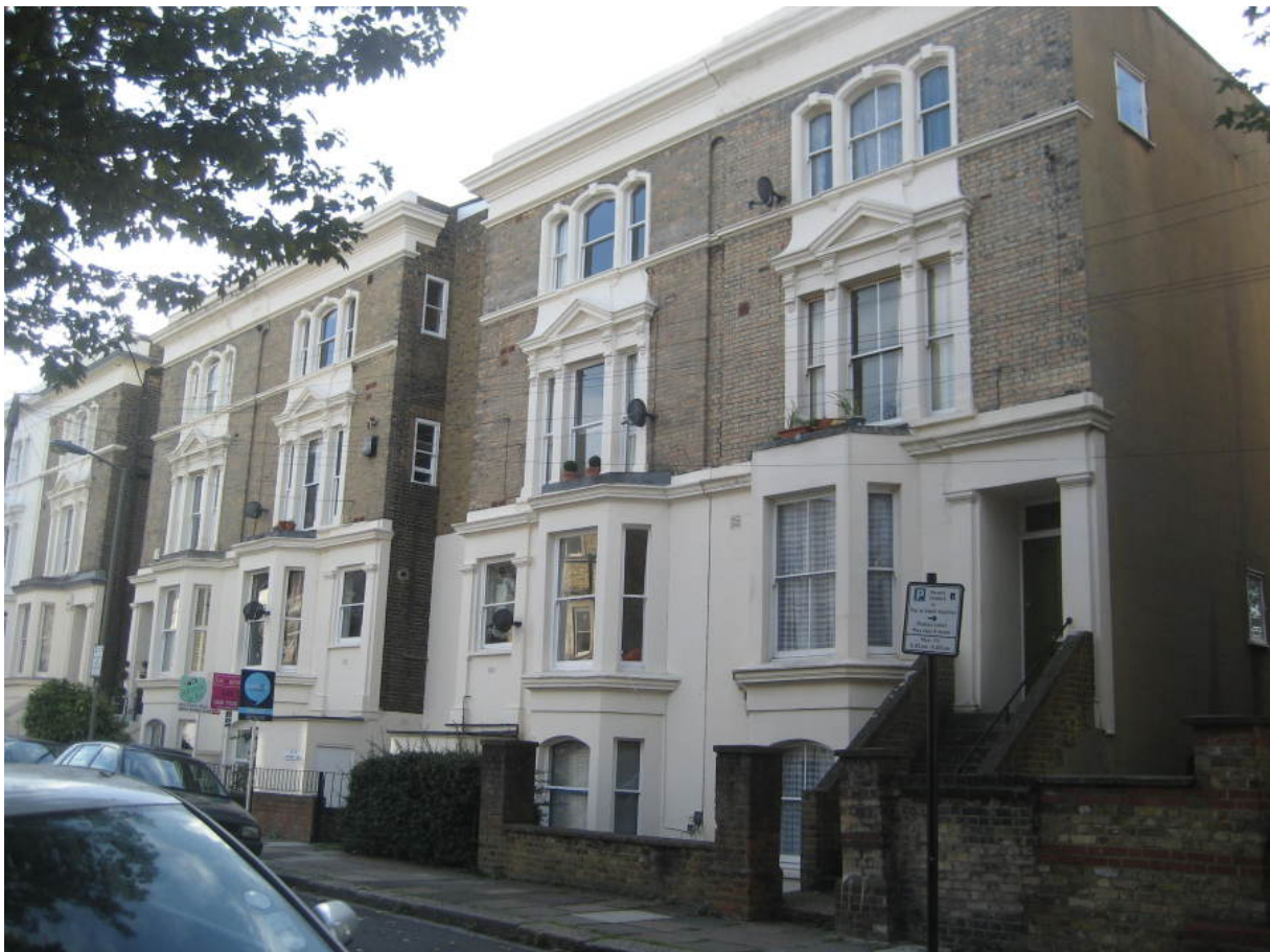
Figure 49 Nos. 7-16 Louvaine Road
