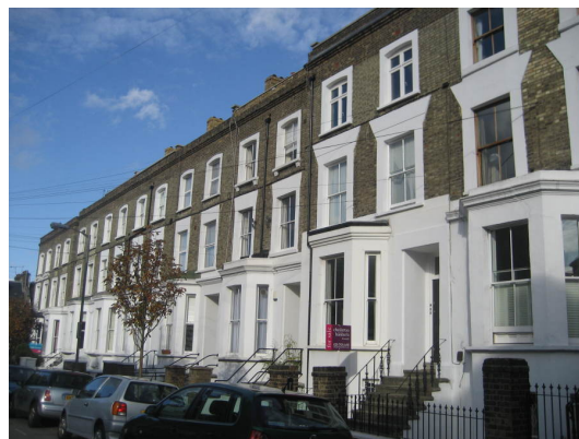
Figure 46 Brussels Road west side
