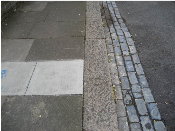
Figure 12 Original scoriier blocks and granite kerbstones with sympathetic grey paving blocks
