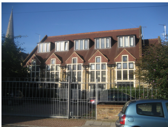
Figure 56 Nos. 6-14 Plough Terrace
