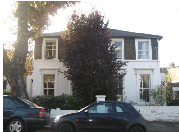
Figure 22 Nos. 33-35 - one of pairs of villas
