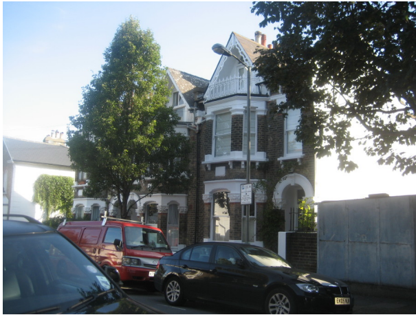
Figure 27 Nos. 2-6 St John's Hill Grove. Houses with unusual gable and balcony
