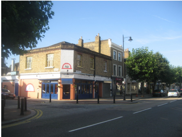
Figure 35 Varying building heights after the Spencer Road junction
