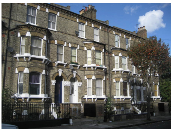
Figure 47 Three storey terrace with basements and original railings
