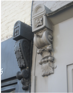
Figure 42 Original console brackets at fascia level
