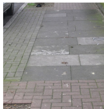
Figure 11 Modern red blocks in a basket weave pattern repair the broken paving slabs and grey blocks have taken the place of grass verges leading to a patchwork appearance.
