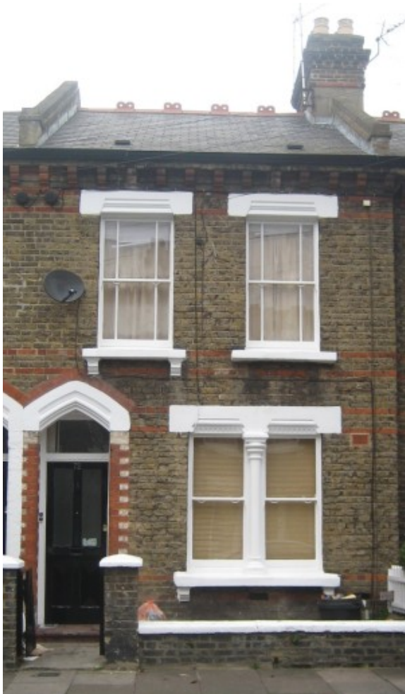
Figure 25 A typical terrace house with original sash windows, slate roof, front door and boundary wall.
