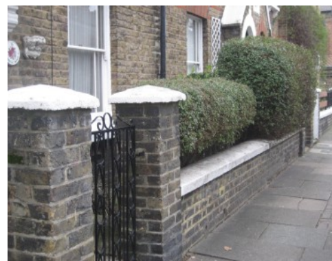
The best solution where railings have been lost: a low wall with coping stone and hedging
