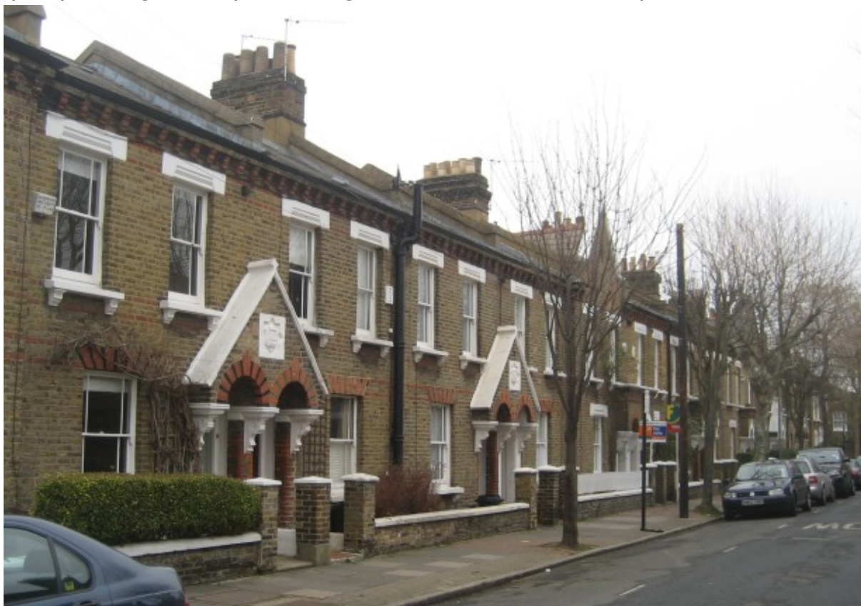
Figure 17 A typical terrace in Sabine Road
