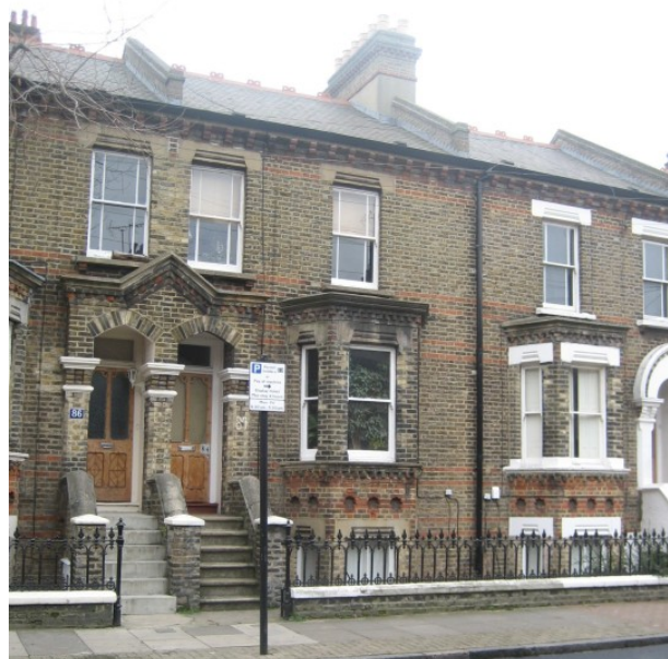
Figure 19 Houses with basement on Grayshott Road
