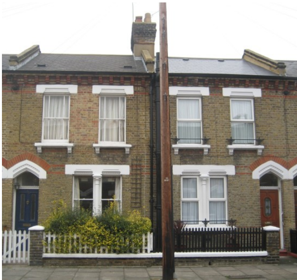
Figure 28 The house on the right has upvc windows which open outwards. They have no glazing bars and their frames are much thicker than the original sash windows as seen in the house on the left. The front door is also a modern unsympathetic design
