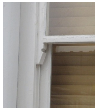
Figure 27 A horn with a straight side and half round notch - typical of the Shaftesbury Park Estate
