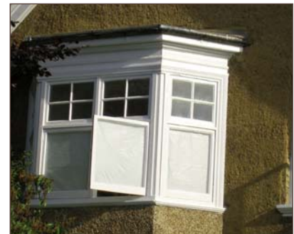
Bay windows with timber casements, decorative mullions and toplights.
