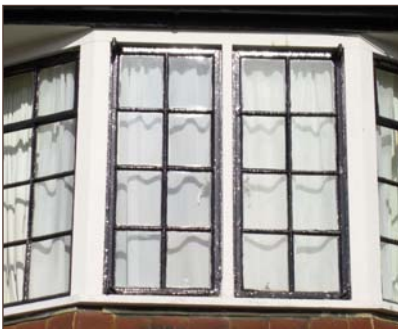
Bay windows with Crittall casements along Lytton Grove.
