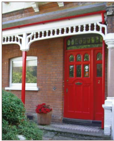
Timberwork recessed porch.
