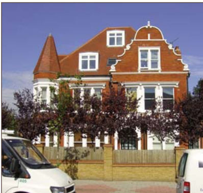
Example of a large detached villa built upon a corner site with Turreted bay window, Dutch gable and dormer windows.
