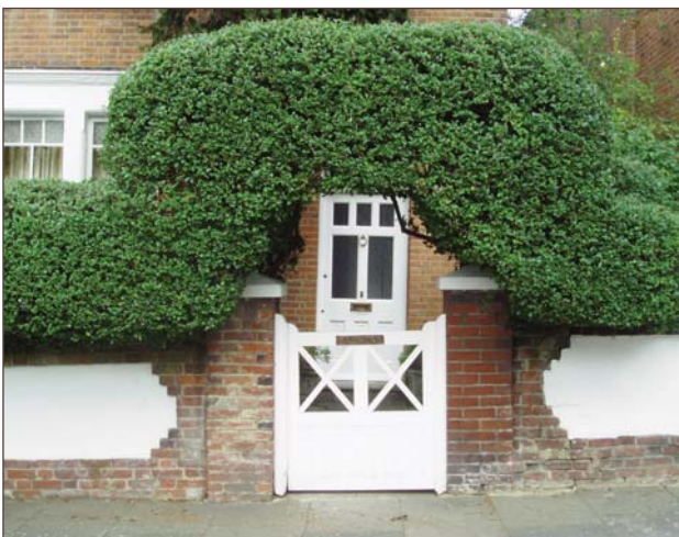
Original brick boundary wall with gateposts with moulded tops and privet hedge.
