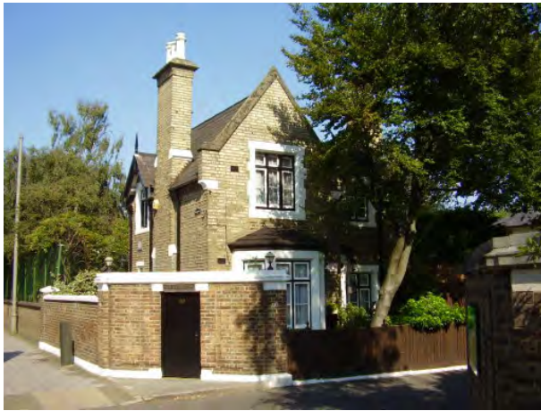
Figure 25 Former gatekeeper's cottage
