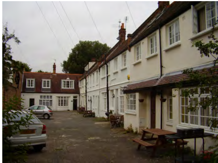
Figure 48 Bensbury Close. Former stables with concrete stable blocks (modern)
