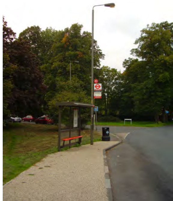
Figure 55 Bus stop with bonded gravel pavement
