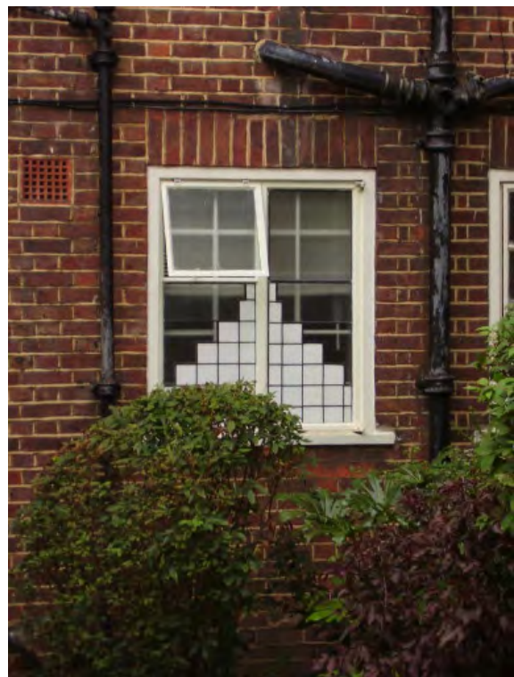
Figure 79 Typical bathroom window to rear of flats
