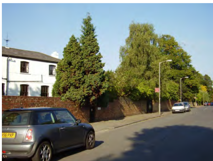
Figure 41 Bowling Green Cottage appears apart from the rest of the street
