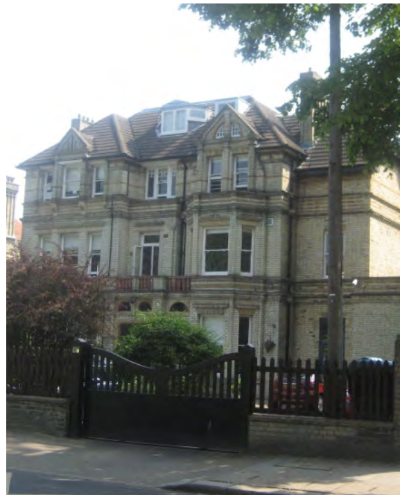
Figure 36 : Prospect House School, 75 Putney Hill
