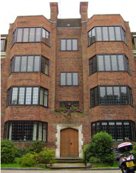
Figure 69 A typical part of one of the blocks with splayed bays and windows with square leading and stained timber frames
