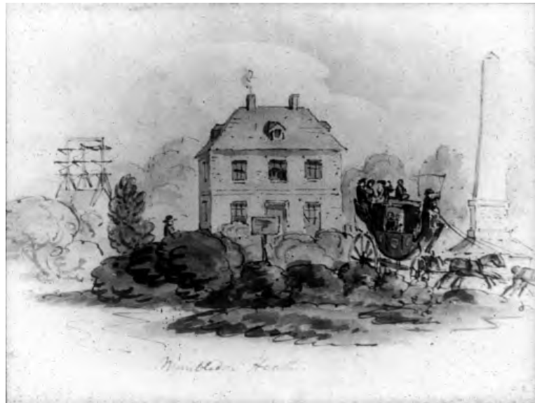
Figure 3 The fireproof house (shown on the 1869-74 map, close to the Telegraph pub) with the telegraph's shutter system on the left of the picture. The obelisk shown remains today
