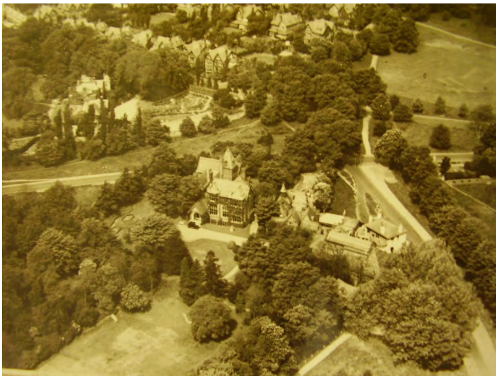
Figure 14 This aerial photograph taken around 1925 shows the Victorian mansion, Wildcroft and its gardens with the Telegraph pub to the right and the newly built houses on Bristol Gardens and Heathview Gardens to the north
