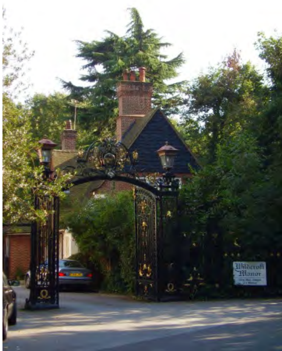
Figure 78 Entrance gates. These are Grade II listed
