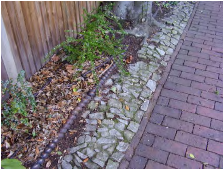
Figure 42 Unusual and highly distinctive paving detail found in this character area
