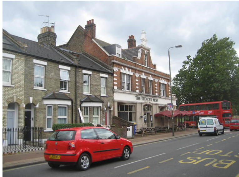
Figure 13 Spencer Arms and the terrace on Lower Richmond Road
