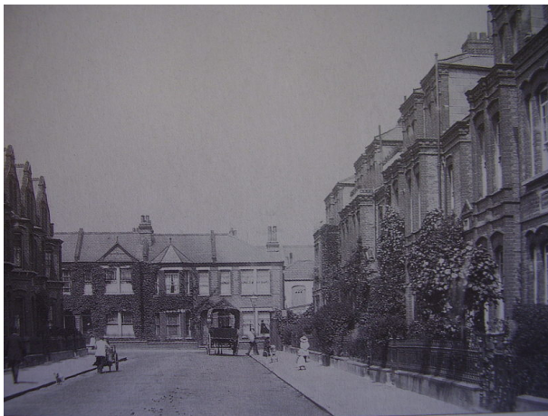
Figure 49 : This photograph taken in 1906 shows the design of the original railings that have since been lost
