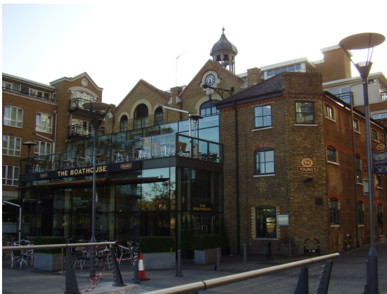
Figure 17 : The Boathouse public house
