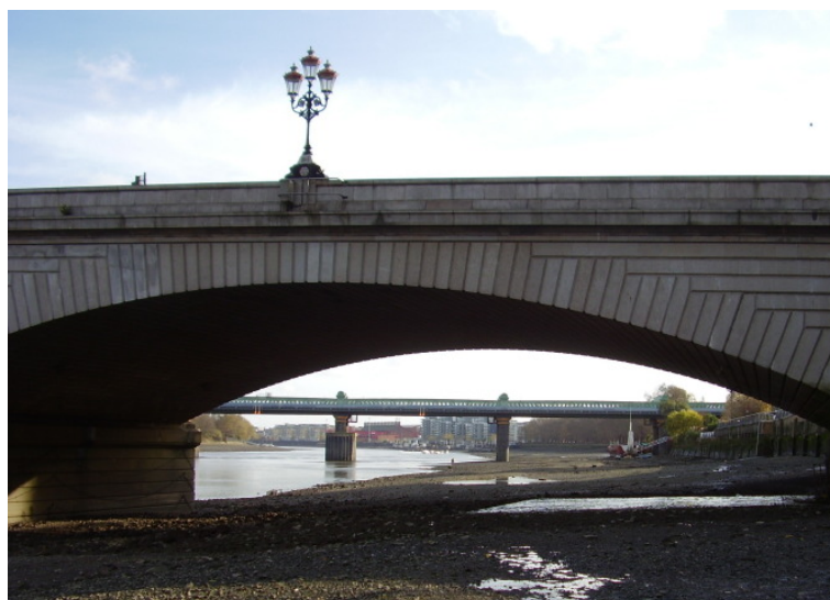
Figure 28 : View through the granite Putney Bridge (for vehicles and pedestrians) to the cast iron Putney Railway (and pedestrian) Bridge in the distance
