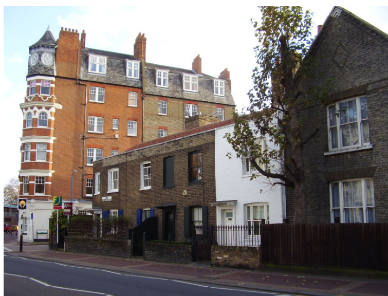
Figure 39 : Cottages at nos. 37-41. No. 43 is seen on the right
