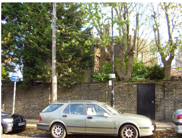
Figure 50 : The wall forming the boundary to Winchester House, seen from Ruvigny Gardens
