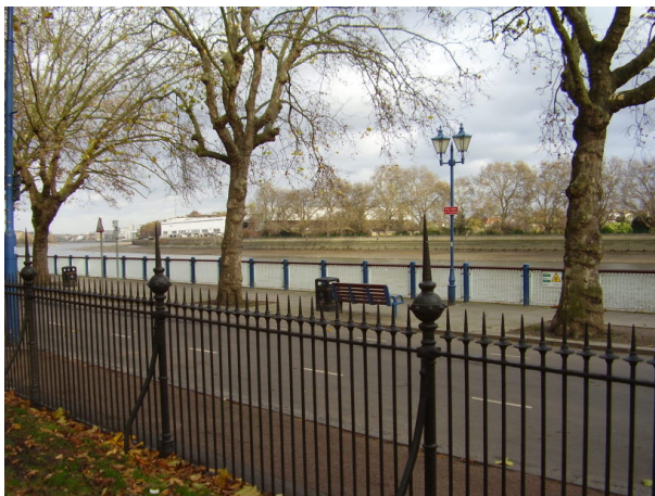
Figure 69 : Park railings with spikes still in place
