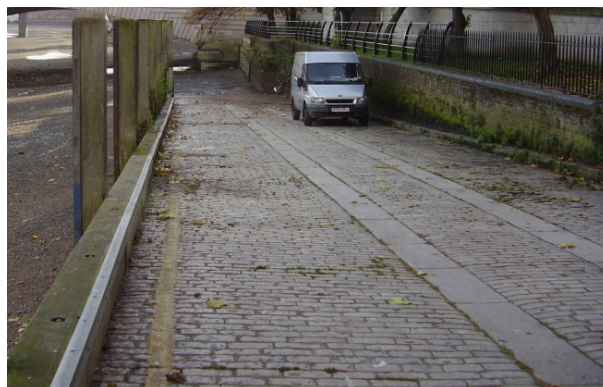
Figure 42 : The granite slipway
