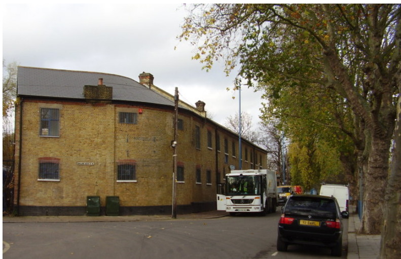
Figure 66 : Sea Cadet Corps building single-storey structure in matching brick added to the rear.
