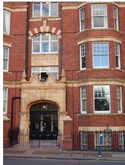
Figure 35 : Terracotta entrance to Kenilworth Court
