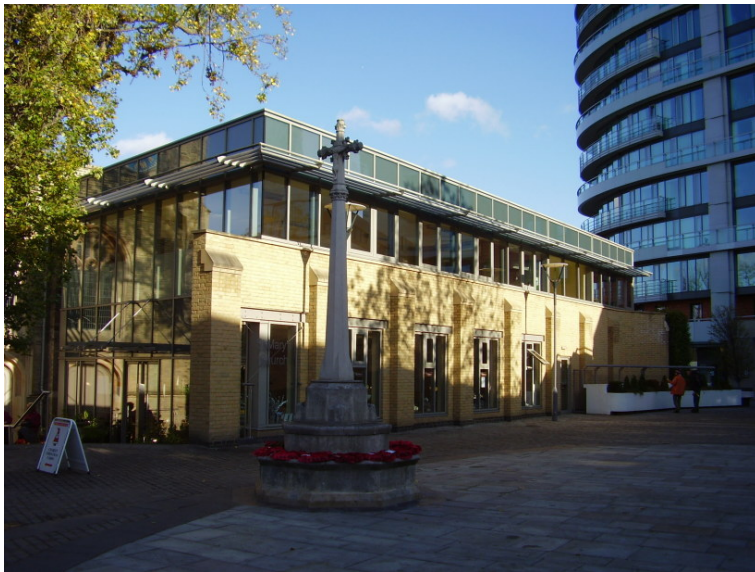
Figure 16 : Community hall extension to St Mary's built in 2006
