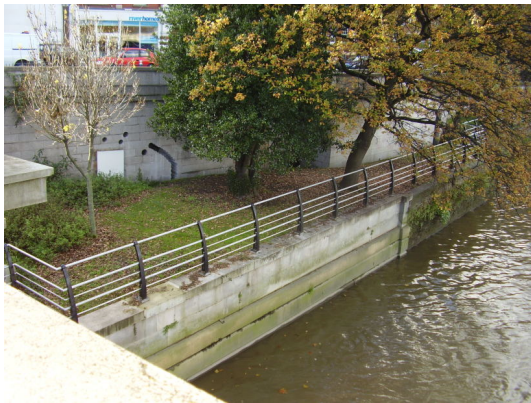
Figure 40 : Flanking wall to Putney Bridge
