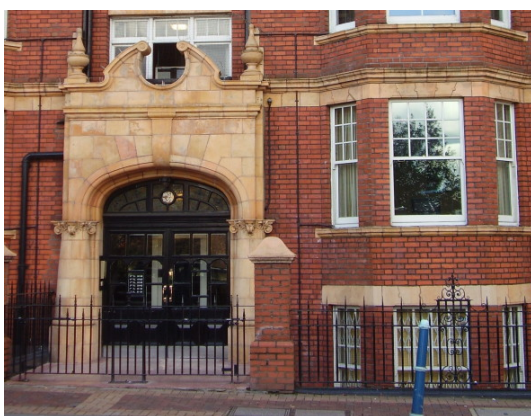
Figure 41 : Railings at Kenilworth Court
