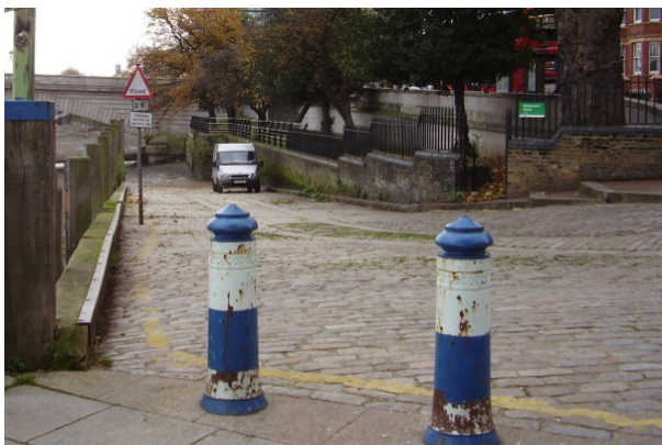
Figure 44 : Victorian cast iron bollards
