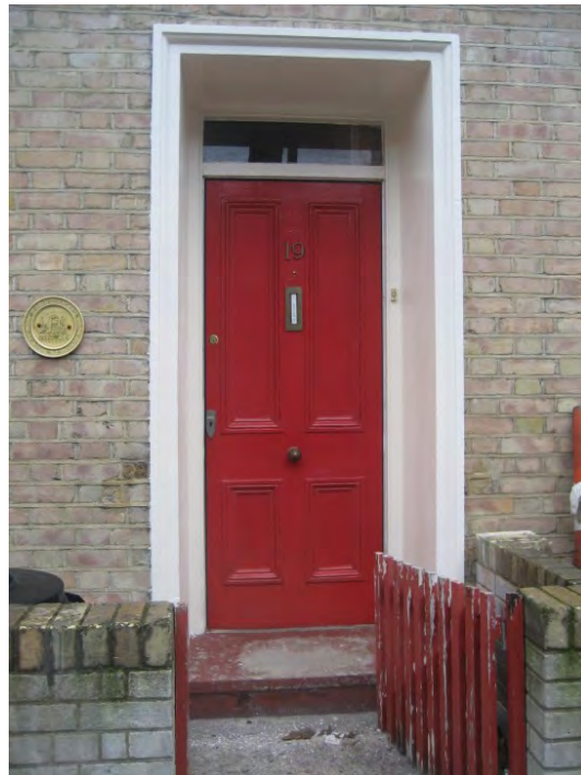
Figure 9 : Four panelled door - typical of the early houses in Park Town
