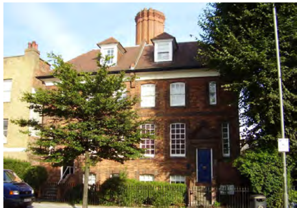
Figure 43 : Nos. 118 - 120 Queenstown Road
