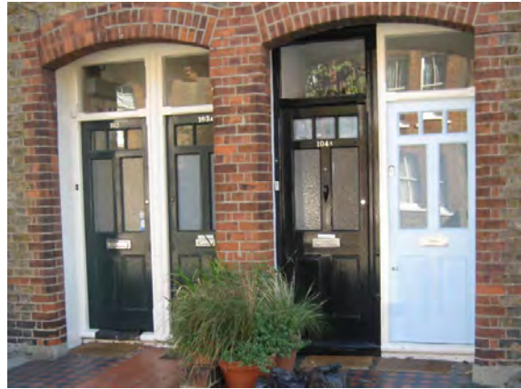
Figure 24 : Two pairs of original doors the flats on Tennyson Street
