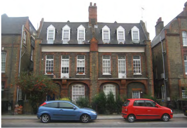
Figure 40 : Nos. 106 - 108 Queenstown Road
