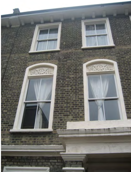
Figure 8 : Sash windows with single glazing bar and stucco detailing above
