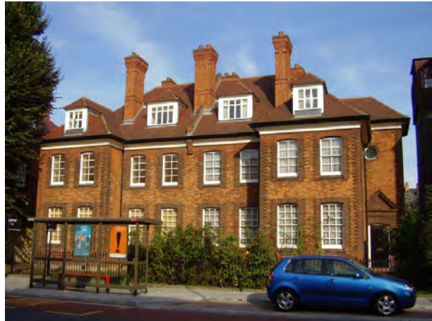
Figure 42 : Nos. 114 - 116 Queenstown Road
