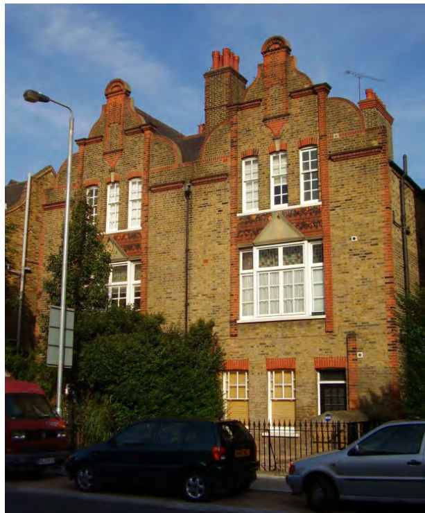
Figure 39 : Nos. 102 - 104 Queenstown Road
