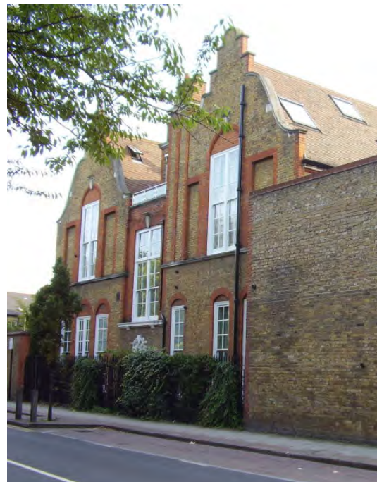
Figure 22 : Later school building by T. J. Bailey (built between 1895-1916)
