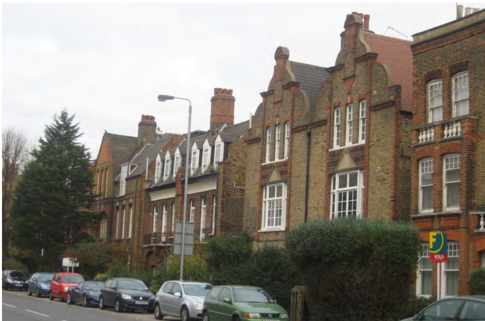
Figure 20 : Houses by T. J. Bailey on Queenstown Road
