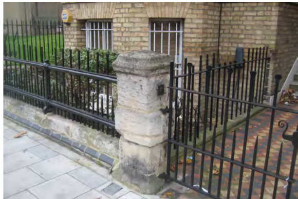
Figure 31 : Original railings and stone pillar seen at nos. 131 and 145 Queenstown Road
