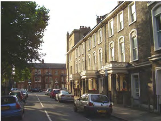
Figure 12 : St Philip Square - southern side
